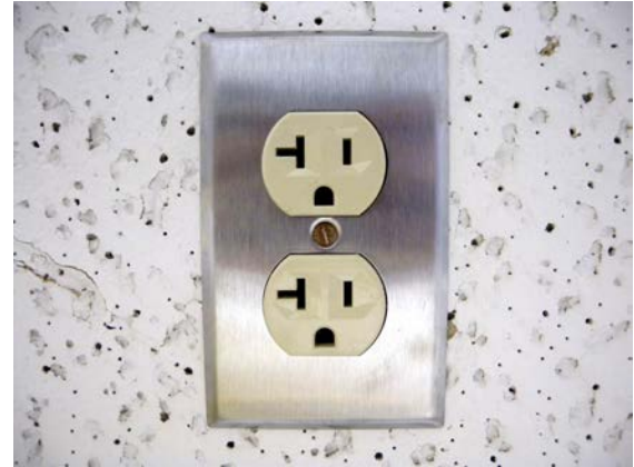
Figure 1-3. NEMA 5-20 outlets feature a horizontal slot for a 20 Amp plug.
