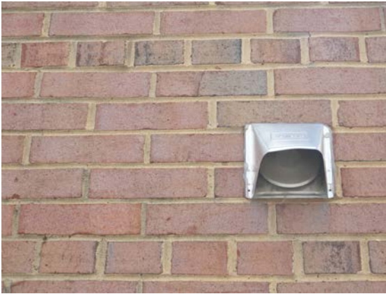
Figure 1-5. The ventilation system directs unwanted fumes outside of the building.
